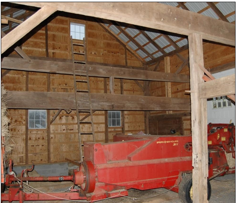
Top: View of Hammerstone Barn in Holland Township, NJ Bottom: Interior View of Swing Beam and Other Framing Members, Hammerstone Barn. Photo Credit: C. Cielo.
