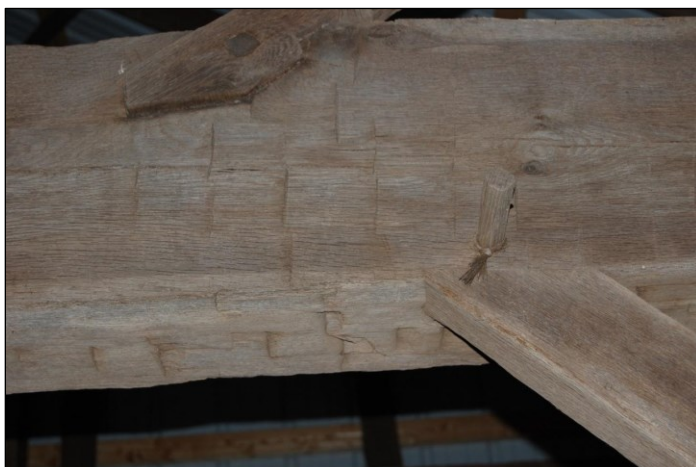
Detail of Bracing Joints at Swing Beam (left) and of Sample Extraction (below). Photo Credit: C. Cielo.
