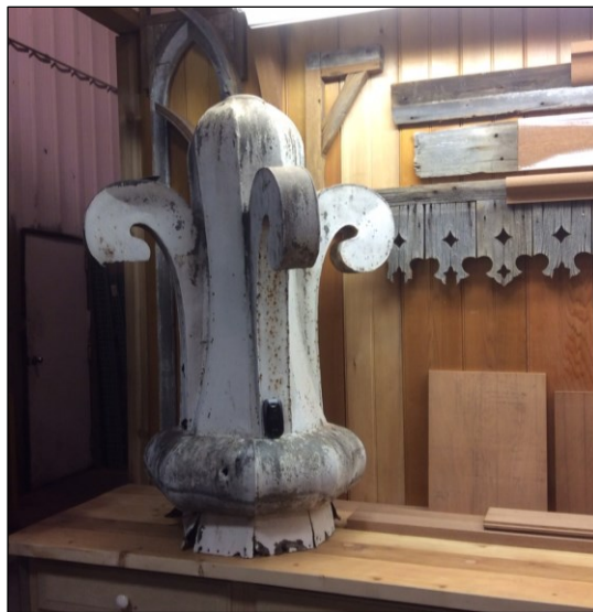
Images from the DAS workshop: At top left, restored cupola for an outbuilding; at bottom right: louvered cupola from hog barn undergoing repairs; at right, original metal fleur-de-lis finial from cupola of Star Barn (note flip phone for scale). Photographs courtesy of Charles Leik.
