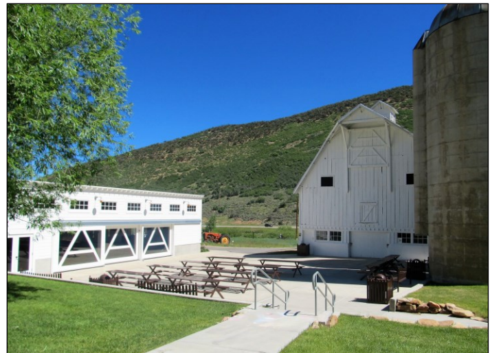
McPolin Farm Farmyard (2 photos) –Today, the original farmyard provides a public gathering space. In 1999, Osguthorpe's open-air shed was demolished and a new event space was constructed in its location adjacent to the farmyard.
