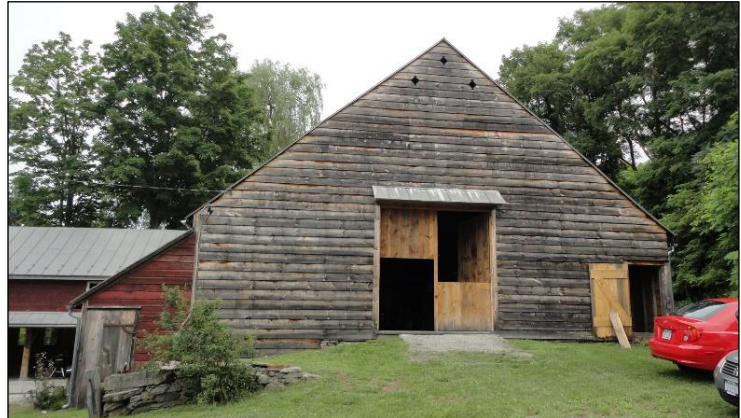
Above: Rodgers Barn, Wappingers Falls, NY, is an original 1790 barn with a 1830 barn (moved whole in the mid-1800s) attached to the rear. This ‘new’ barn was lowered and tilted to make the two ridgelines match. Restoration included Dutch door design from another local barn.
