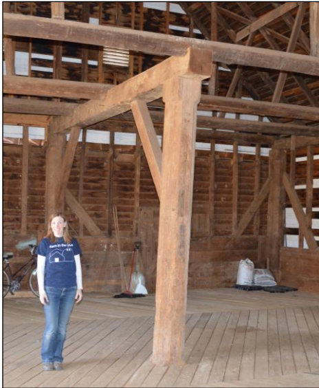
At left, interior view of Clover Hill's English bank barn with NBA Past President, Danae Peckler, acting as scale bar at 5' 7" next to original chamfered posts. At right, detail of Emily Anderson's drawing of post profile.
