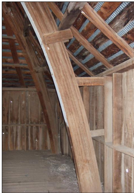
Above: Closer View of Framing System and Section of Rafter. Measurements taken by Byron Ulery indicate that each member of the roof's truss system are roughly 12.5 inches thick and composed of up to 15 sawn boards.
