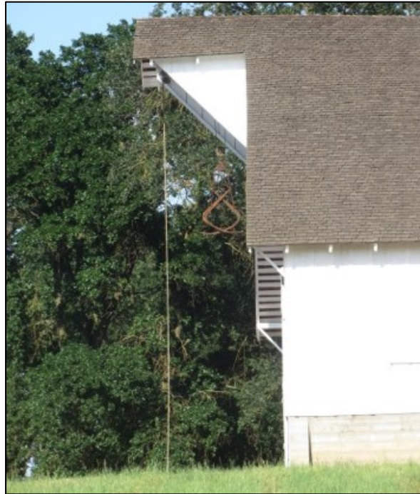
Left: Hayloft Pulley. Top right: Pyramidal bracing extends from the corners to the roof ridge. Bottom right: Side stalls in the Draft Horse Barn at Rancho Omochumnes. Images courtesy of J. Prager.
