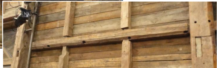
Below & Inset: Detail of Re-Used Barrack Pole
