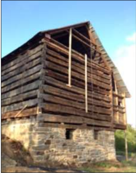
View of southwest corner during work..
