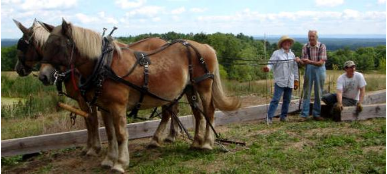
Ev Rau borrows his neighbor's draft horses to pull new sills into place
