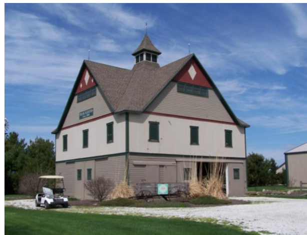
The Flack Barn, 1900, Macomb. This has cross-gable construction, allowing no posts under the central hay mow ventilator.
